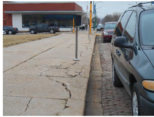
High Curb/Damage – Stone Street – 1500 Block
