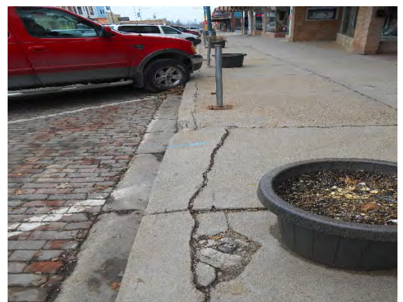
Broken Sidewalk/Curb – Stone – 1600 Block
